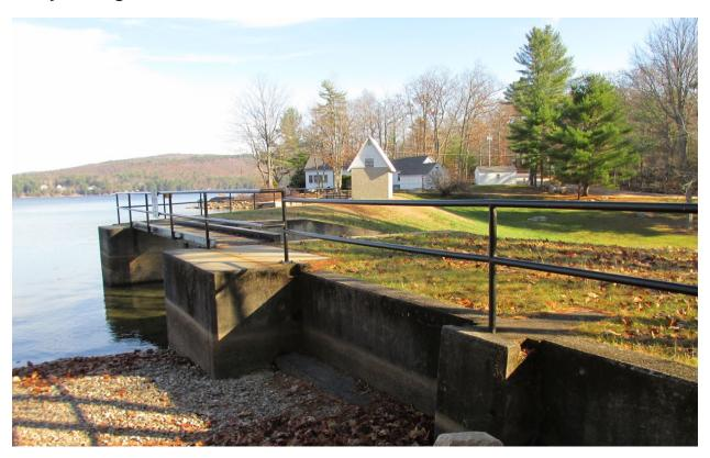
Merrymeeting Lake Dam is a high hazard, earthen embankment dam with a concrete spillway, located in New Durham at the outlet of Merrymeeting Lake. Originally constructed in 1924, it was reconstructed in 1969 and again in 1983. The dam is 285 feet long and 22 feet high, and it is owned by the New Hampshire Fish and Game Department and operated in coordination with the NHDES Dam Bureau. Its primary purpose is recreational water management.
