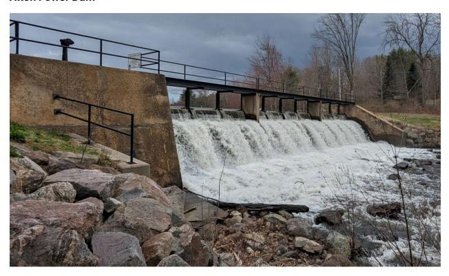
Alton Power Dam is a high hazard, concrete gravity dam located in Alton, New Hampshire. Built in 1923 and rehabilitated in 1979, the dam is 190 feet long and 16 feet high. It is owned by the New Hampshire Fish and Game Department and operated in coordination with the NHDES Dam Bureau. Like the other dams in the watershed, it was originally constructed for hydroelectric purposes and now supports recreational use.
