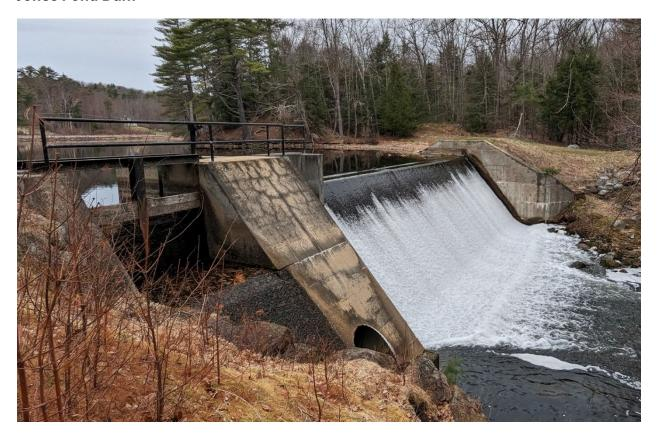
Jones Pond Dam is a high hazard, concrete gravity dam located in New Durham. Constructed in 1924 and reconstructed in 1986, the dam is 210 feet long and 21 feet high. It is owned by the New Hampshire Fish and Game Department and operated in coordination with the NHDES Dam Bureau. The dam was originally built for hydroelectric power generation and now serves recreational purposes.
