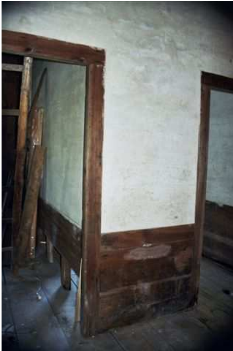
1830-40s door casings located at doorways to small front rooms and vestibule
