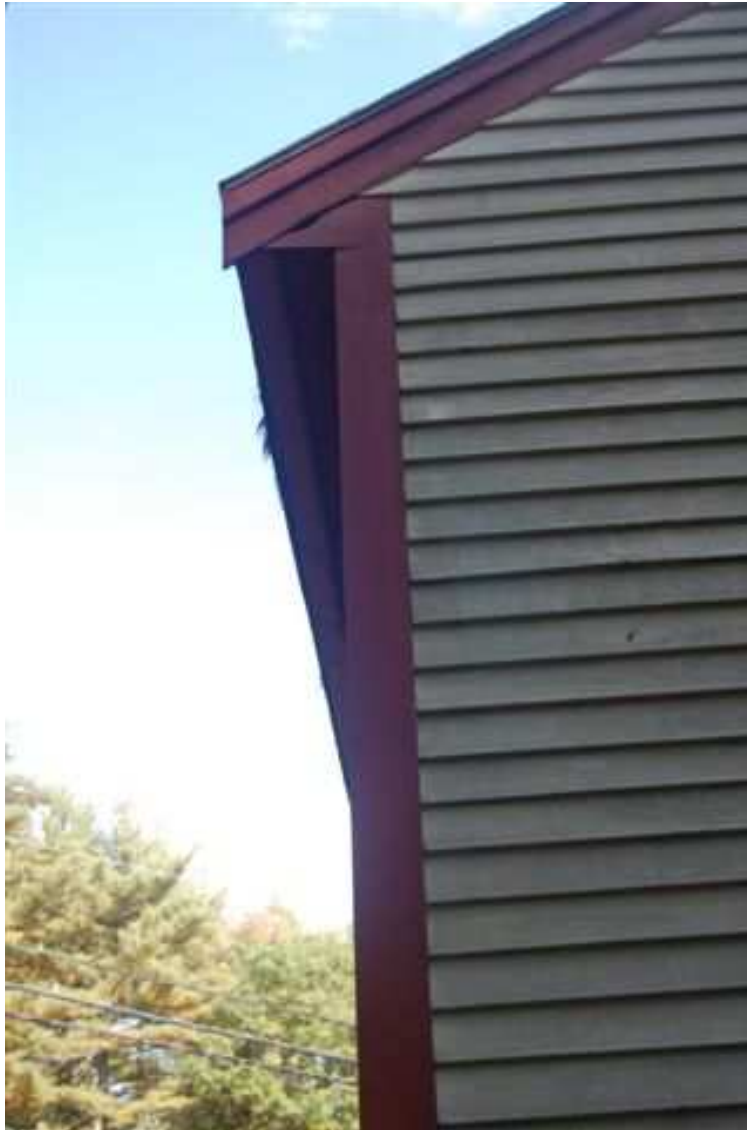
Detail of replacement siding and trim
