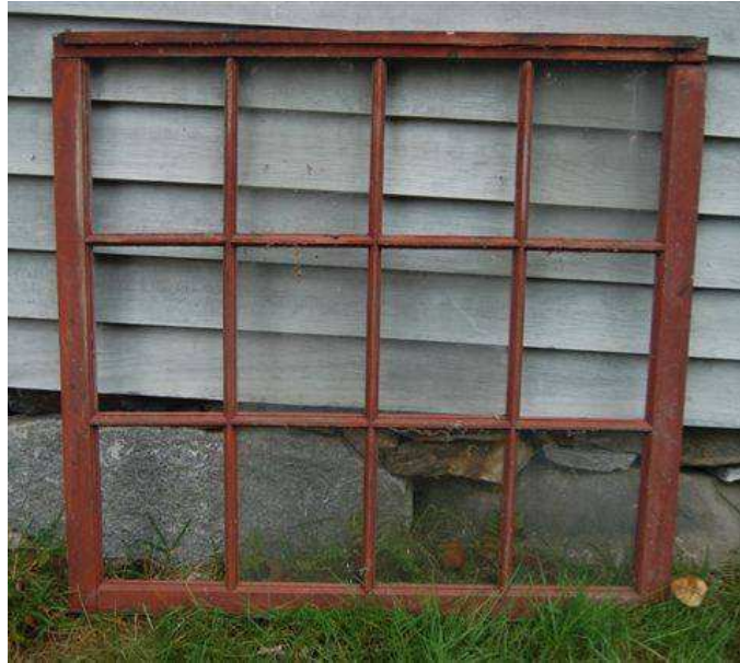
At left: detail of a replacement window. At right: sole surviving historic sash, likely from the 1791-92 era
