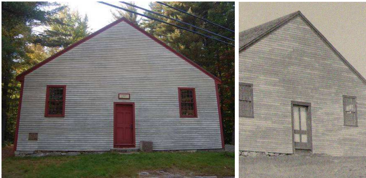
Front (northeast) elevation. From the mid-19 th c. until the late 1980s, the front door had four panel. (at right: detail of a late 19 th century photograph in the collection of New Hampshire Historical Society)
