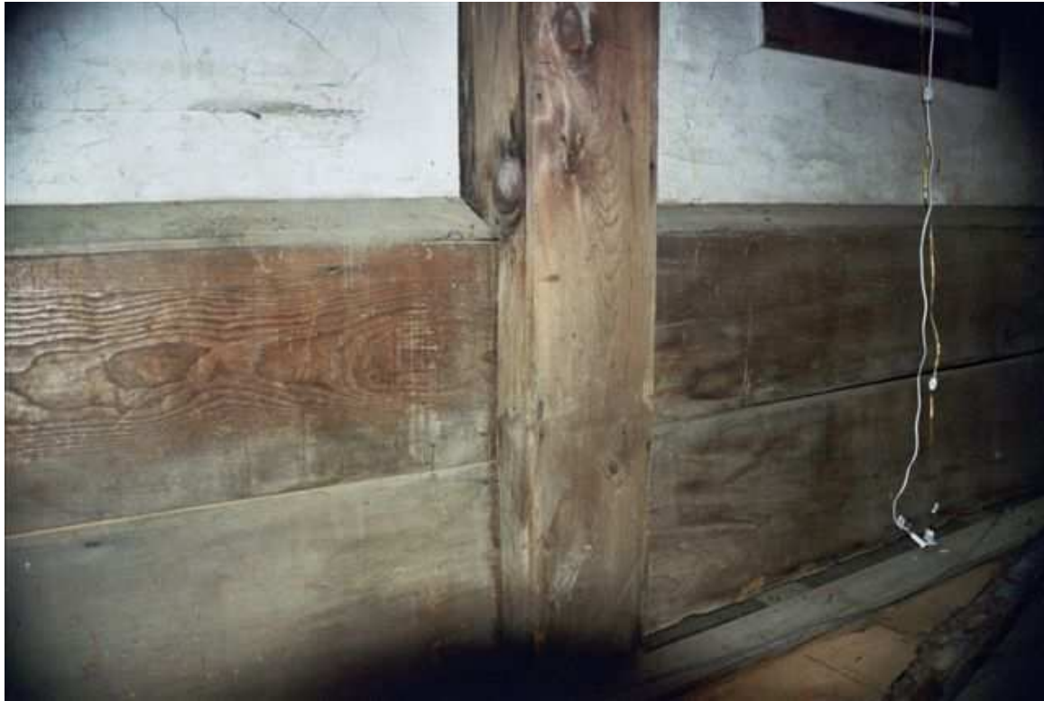
Detail of 1792 wainscot, showing also the 1838-1847/48 wainscot cap and post covers.
