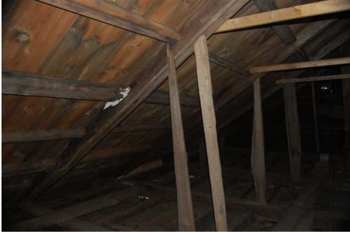
Roof framing system, showing original (1769) hewn rafters and purlins. The white patch shows an area that had gotten wet and may need to be repaired (or replaced with like material if it is not salvageable). The left vertical brace is one that was added to keep the collar tie from sagging. The sheathing boards seen in this photograph are replacements.
