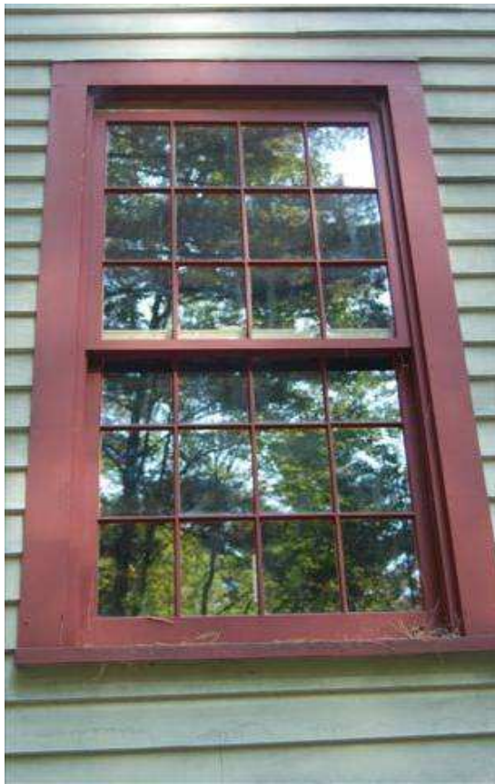
At left: detail of a replacement window. At right: sole surviving historic sash, likely from the 1791-92 era
