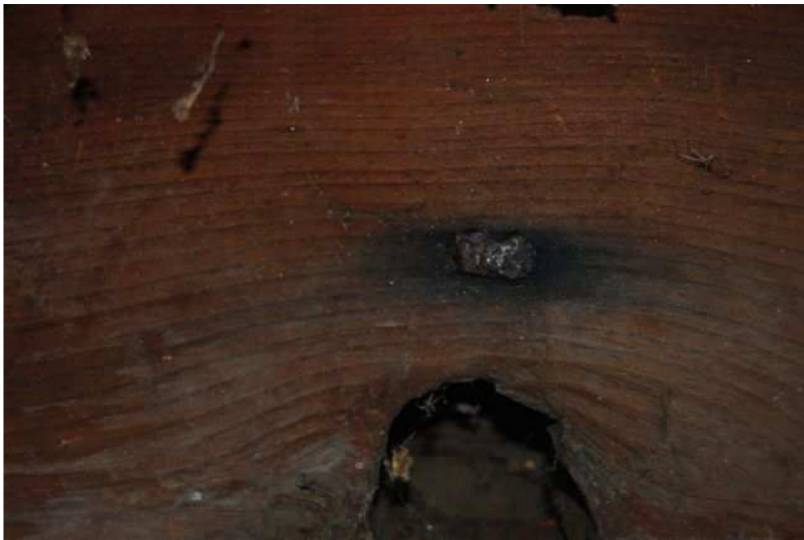
18 th c. butterfly wrought iron nail found in wainscot
