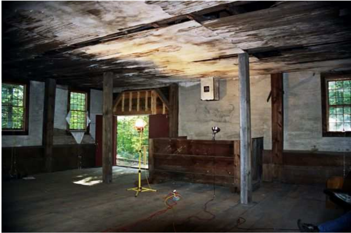
Interior view showing moderator's box at center. Interior posts are not original.
