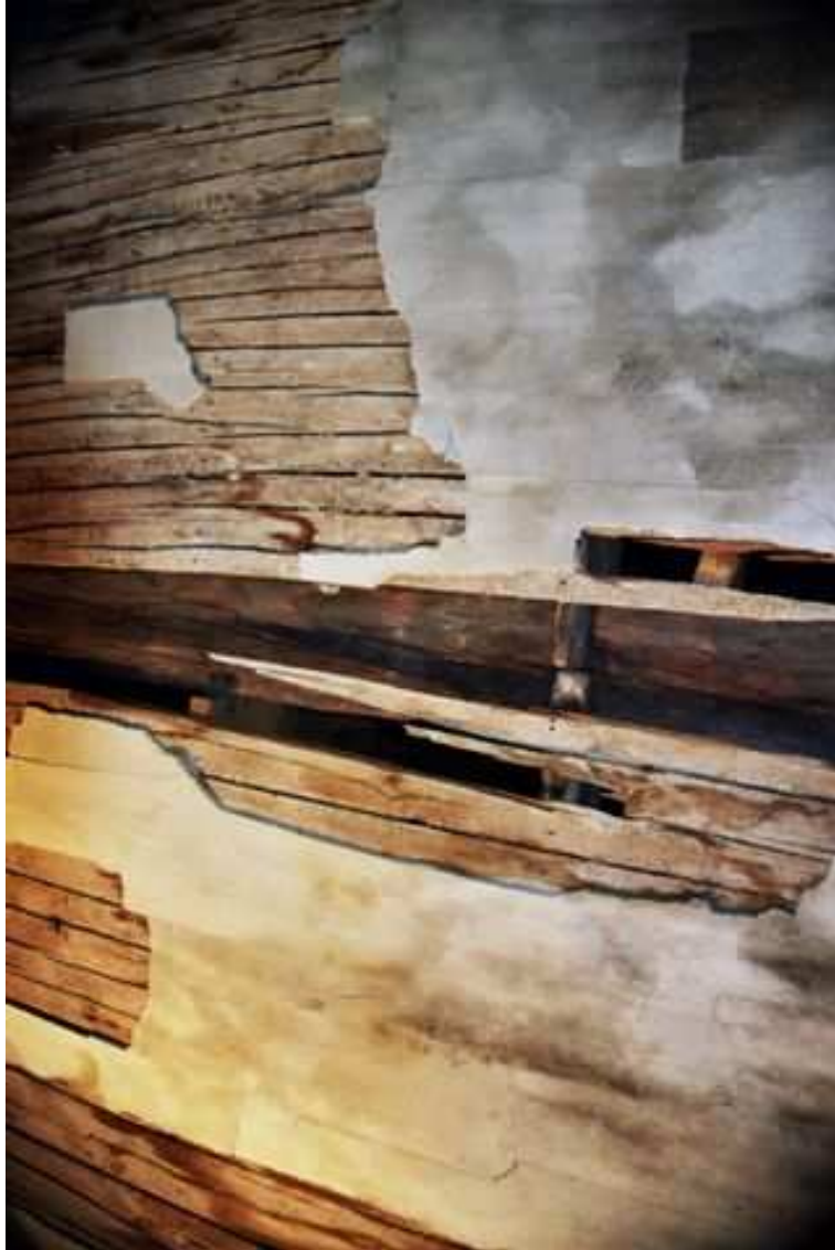
Detail of split/accordion lath on walls
