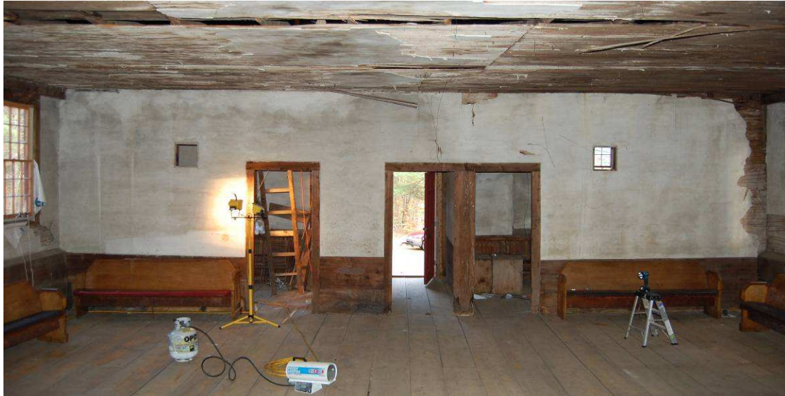
Looking northeast toward the two small rooms at the front of the building. The square openings once held stove pipes connecting the stoves in the small rooms with the chimney on the southwest wall.
