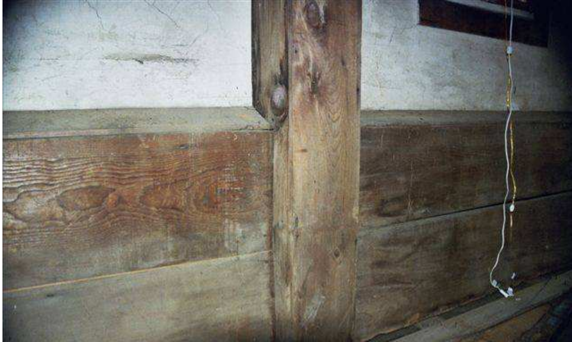
A section of the first floor wall showing wainscot with cap and a covered post
