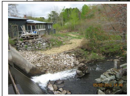
Downings Dam Work
